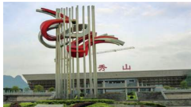
Chongqing Xiushan Railway Station and Supporting Works
