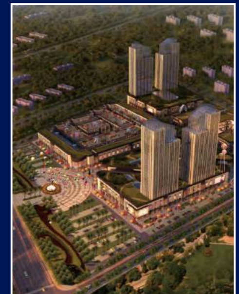
Phase II of the Zhong'A International Trade City, Jinji Town, Wuzhong City, Ningxia
