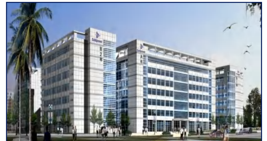
Shenzhen Goldpower Technology Industrial Park
