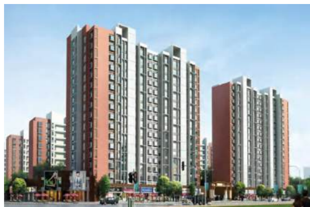
Phase I of Wangqian International City, Laohekou City, Hubei Province
