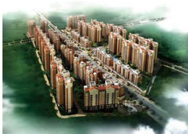
Jinpu Huayuan, Pubei County, Qinzhou City, Guangxi Province
